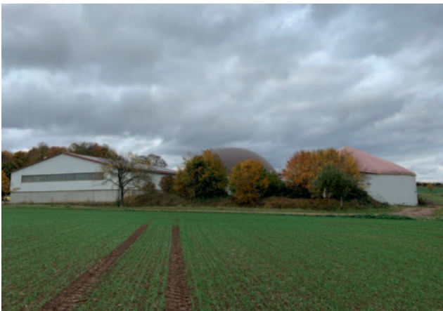
Biogasanlage Fa. Rube
